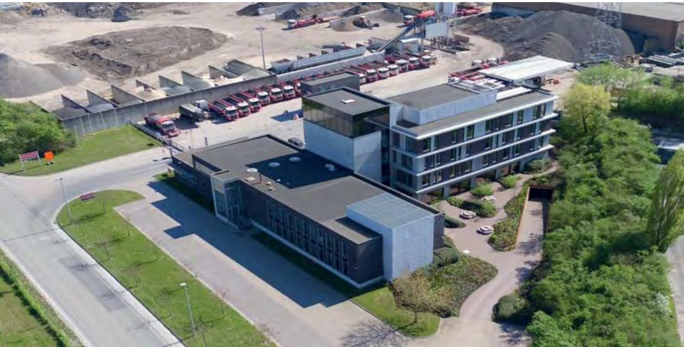
Figure 4: Stadsbader office building
